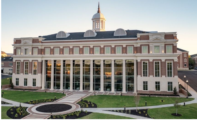
Front entrance to Jones Hall College of Health Sciences. Photo courtesy of Today.Troy.edu
